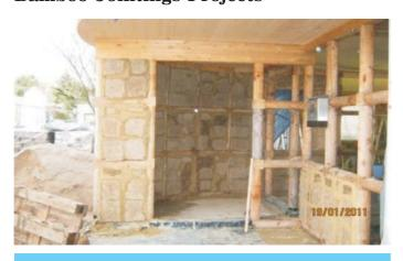
NMBA has supported technology for development of bamboo jointing with whole bamboo and using local material for construction of multi-storey houses. This is based on German Technology and the project is being implemented in Arunachal Pradesh.
