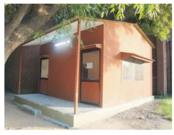
NMBA has been engaged to set up engineered bamboo based structures to be used for various purposes like class room and canteen in various colleges of Delhi University. These have been well received by the university authorities and have created a good response from South Campus, Delhi University vistors. NMBA is now erecting structures of size 28'x20' & 16'x16' for Kamla Nehru and Maitreyi and Gargi College, respectively.
