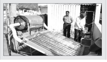
This solar heater developed by Shri S B Janakiraman of Vellore. made use discarded fused tube lights and other waste materials. It has a tank capacity of 100 litres to 200 litres. A temperature of about 60-65 °C is achievable within 3 hours, if the initial ambient temperature is about 30 °C. As it makes use of discarded fused tube lights, this solar water heater provides cheaper water heating options for households, hostels, small offices, workshops, hospital rooms etc.
