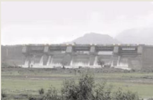
*Replacement of 65% cement by Fly Ash- Upper dam of Ghatghar pumped storage scheme (Near Nashik, Maharashtra constructed with Roller Compacted Concrete technology*
