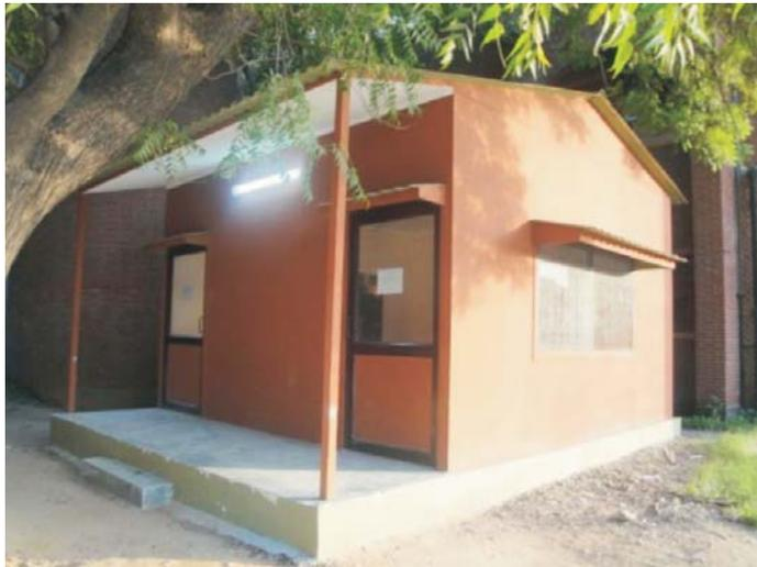
NMBA has been engaged to set up engineered bamboo based structures to be used for various purposes like class room and canteen in various colleges of Delhi University. These have been well received by the university authorities and have created a good response from South Campus, Delhi University visitors. NMBA is now erecting structures of size 28’x20’ & 16’x16’ for Kamla Nehru and Maitreyi and Gargi College, respectively.
